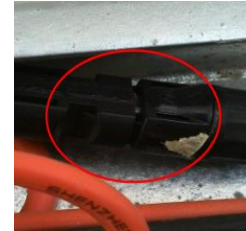
The cable is loose
